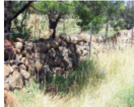
Dry Stone Wall C49
