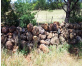
Dry Stone Wall C49
