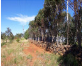
Dry Stone Wall C50
