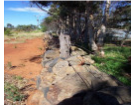
Dry Stone Wall C50
