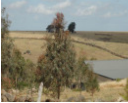
Wall A263 western end - view from Finchs Road
