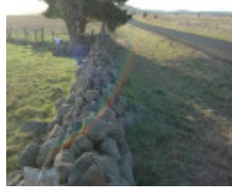
Dry Stone Wall R194
