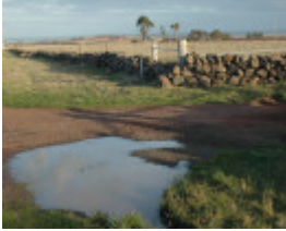
Dry Stone Wall R194
