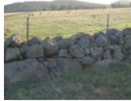
Dry Stone Wall R194
