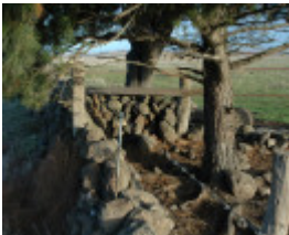
Dry Stone Wall R194
