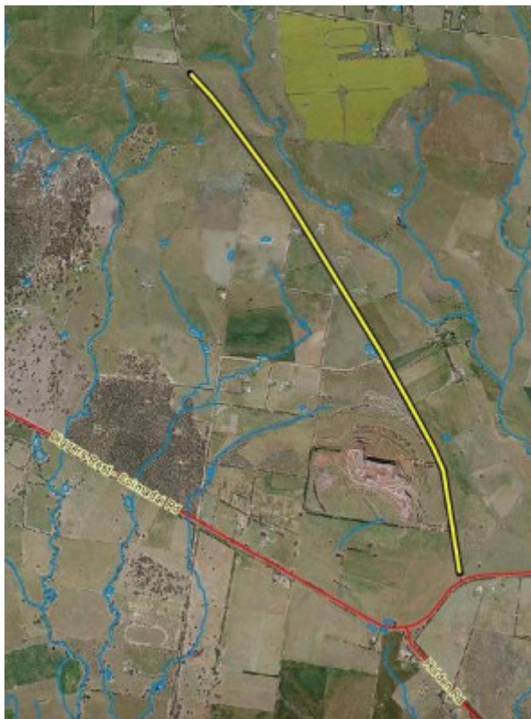
Dry Stone Wall R248
