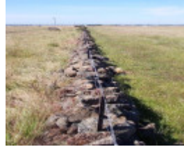
Dry Stone Wall G84
