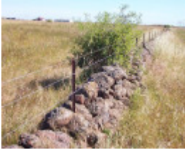
Dry Stone Wall G84
