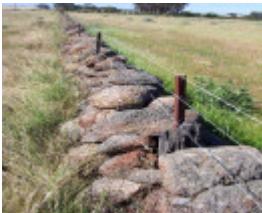
Dry Stone Wall G84
