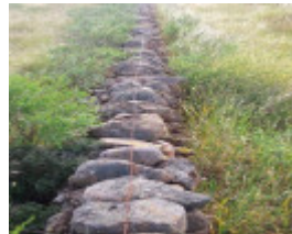
Dry Stone Wall C69
