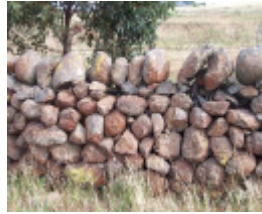
Dry Stone Wall C69
