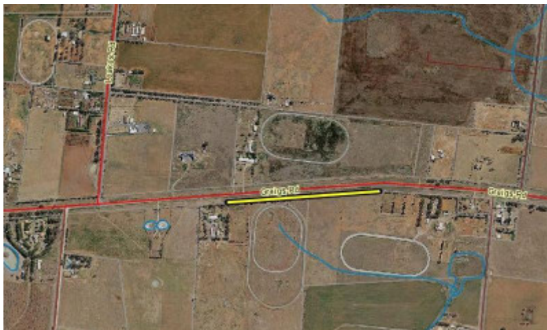
Dry Stone Wall C69
