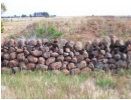
Dry Stone Wall C69
