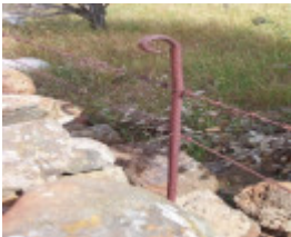
Dry Stone Wall C69
