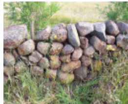
Dry Stone Wall C69
