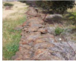
Dry Stone Wall C69
