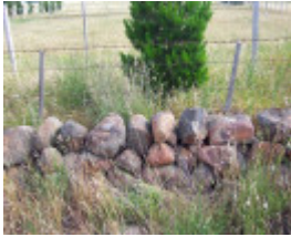
Dry Stone Wall C70
