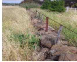
Dry Stone Wall C70
