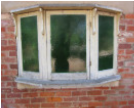
48-56 Taylor Street, detail of window added c.1920
