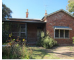
48-56 Taylor Street, front elevation showing projecting gable addition
