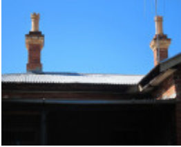
48-56 Taylor Street, chimney detail
