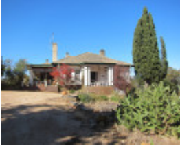
125-133 Mclvor Road, porch & main entry
