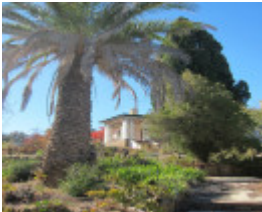
125-133 Mclvor Road, palm tree & entrance porch
