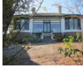
125-133 Mclvor Road, frontage overlooking garden
