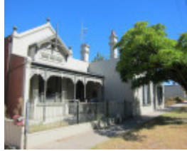
89-91 Lucan Street, residence on left & shop on right
