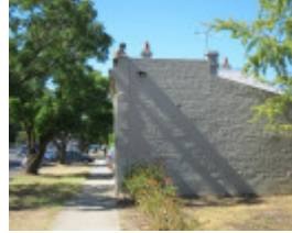
105 Lucan Street, side view
