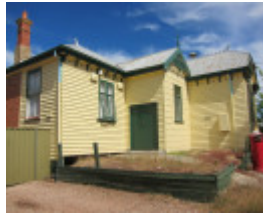
532 Napier Street, former White Hills Reading Rooms & Free Library (2)
