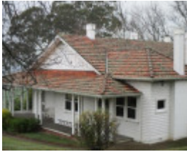
Weatherboard Farmhouse (H12)
