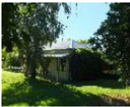
Photo 4: Newtown Brae, single storey addition built in 1885, February 2016.
