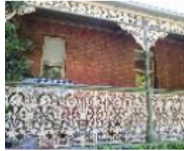
Photo 3: Newtown Brae, detail of east elevation showing delineation in the brickwork (centre) of the original dwelling (right) and single storey front addition (left), February 2016.
