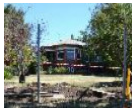
Photo 8: 'Minnewanka', 1 Stephen Street, north (rear) elevation viewed from Formosa Street, November 2015.
