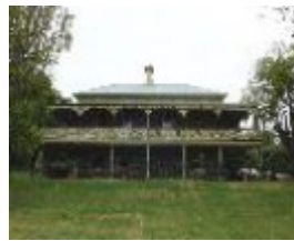
Photo 5: Newtown Brae, two storey addition built in 1885, March 2014.
