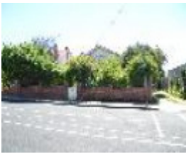
Photo 25: Front fence, 112 Aphrasia Street, November 2015.
