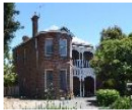
Photo 6: Brooklyn, principal (east) elevation, November 2015.
