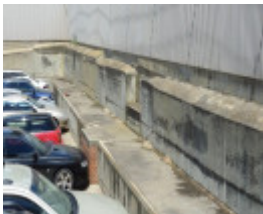
Retaining wall and raised platform (Element 7)
