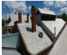
Roof form of Building 6
