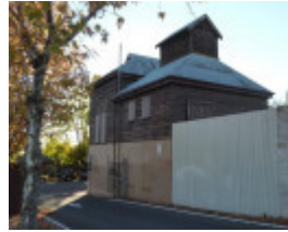
North elevation of the former ice works (corner building, Building 1) and the adjacent fermentation rooms (foreground, Building 2)
