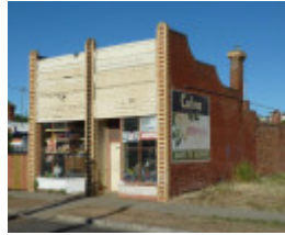
Viewed from the north-east, showing the east return wall
