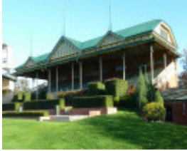
The 1902 Grandstand as viewed from the east
