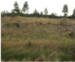
Dry Stone Wall N228 - Internal Wall - North of the Kororoit Creek
