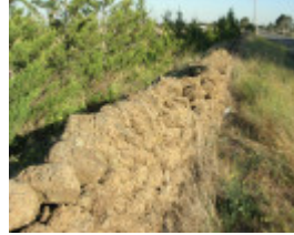
Dry Stone Wall N240 - Sinclairs Road Boundary
