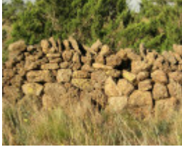
Dry Stone Wall N240 - Sinclairs Road Boundary
