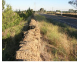
Dry Stone Wall N240 - Sinclairs Road Boundary
