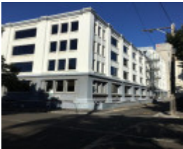
1931 building, view from corner of Little Victoria and Napier streets
