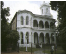
1 cullymont selwyn street canterbury front view
