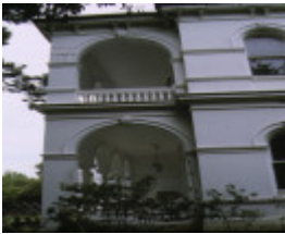
cullymont selwyn street canterbury side view
