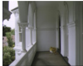
cullymont selwyn street canterbury balcony
