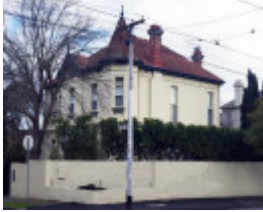
2B Erskine Street, Armadale
