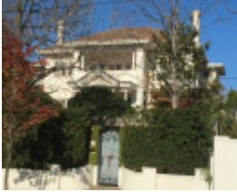
618 Toorak Road, Toorak
