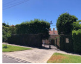
232 Kooyong Road, Toorak
