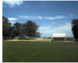
Figure 9: Barrabool Recreation Reserve looking south to the pavilion following alterations, n.d. [c.2014]. Source: Crown Reserve file Rs 4144 DELWP.
