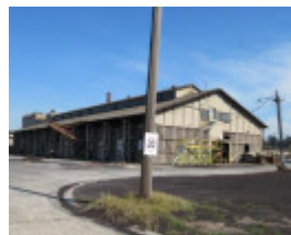
Briquette Storage Shed
