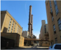
View looking west between Briquette Factories (right) and Power Station with chimneys 3 and 4 (left).
