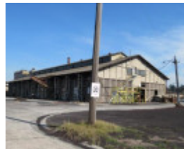
Briquette Storage Shed
