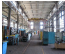
View inside the Mechanical Workshops, looking east.
