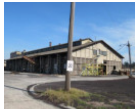
Briquette Storage Shed
