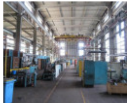
View inside the Mechanical Workshops, looking east.
