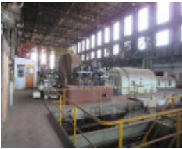
View inside the Turbine House, looking northeast.
