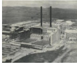
Morwell Briquette Works under construction, 1959.
