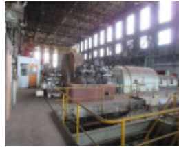
Wet Section Building
