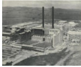
Morwell Briquette Works under construction, 1959.
