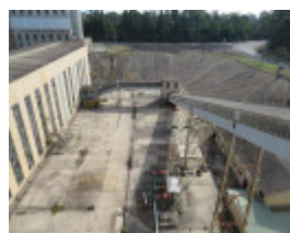
View east from the top of No.1 Briquette Factory looking at the conveyors and North West Corner Station.
