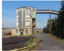
Raw Coal Bunker
