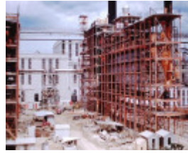
Construction of the Briquette Factories, undated.
