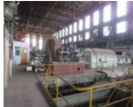
Wet Section Building
