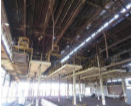
View from under the briquette loading station.
