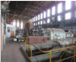
View inside the Turbine House, looking northeast.
