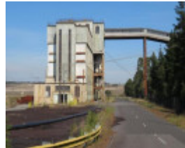
Raw Coal Bunker
