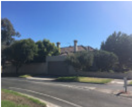
Coburg, 26 Walsh Street (8).JPG
