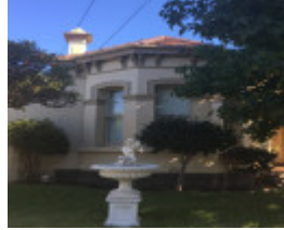
Coburg, 26 Walsh Street (5).JPG
