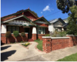
Meaker Avenue Precinct
