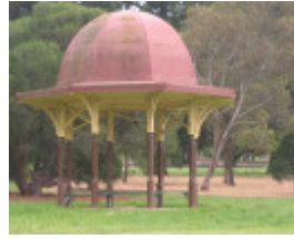
H2095 Eastern Park 29 10.2005 Former Ladies Kiosk
