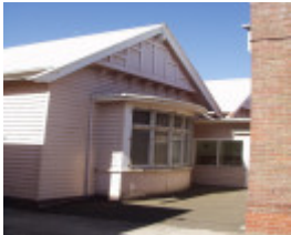
Guild Hall - 33 Myers Street, Geelong - Exterior Rear
