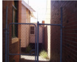
Guild Hall - 33 Myers Street, Geelong - Exterior Side View
