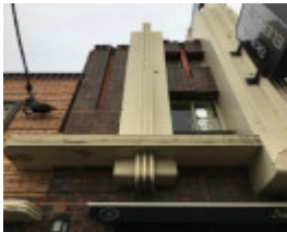
2017 1938 facade detail fins.jpg
