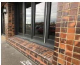
2017 1938 facade window opening.jpg
