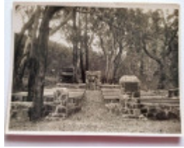
Chapel under construction
