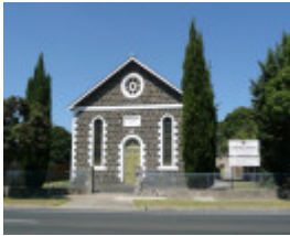
NOBLE STREET UNITING CHURCH, HALL AND KINDERGARTEN SOHE 2008
