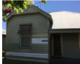
House, 84 Main Street
