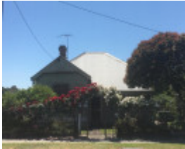
House, 84 Main Street
