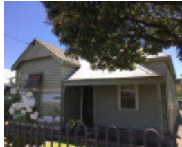
House, 84 Main Street
