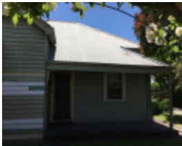
House, 84 Main Street
