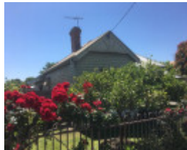
House, 84 Main Street
