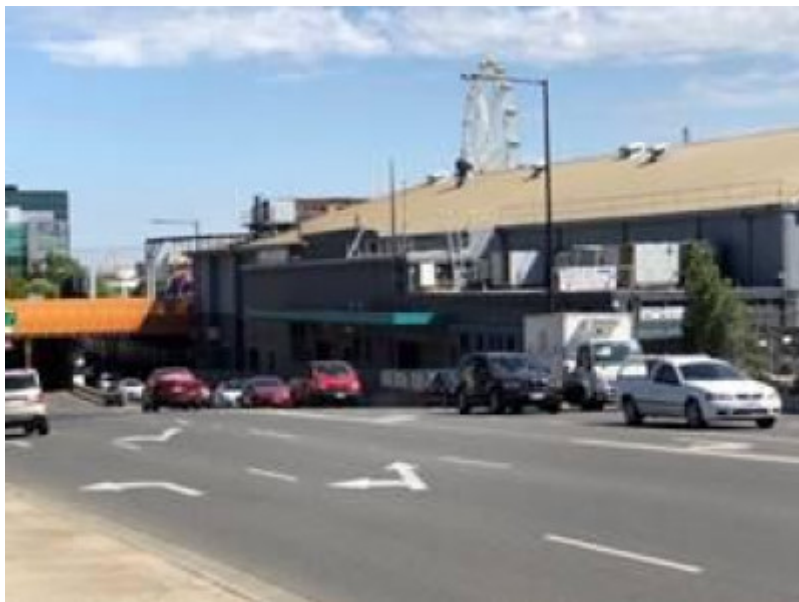
2018, Dudley Street from south-east 2.jpg
