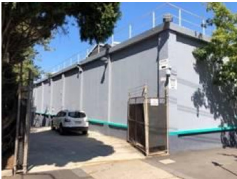
2018, east elevation from north east.jpg
