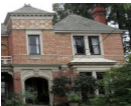
17 Ethel Street Figure 7 Classically inspired cast- cement surrounds to the window and door openings. (Source: Context, 2017) .jpg
