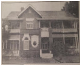
Figure 6. A photo of the house showing the verandah details at this date (SHC, date not known, probably late 20th century).outbuildings and two bungalows to the rear (SCC PF).
