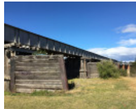
2018, Timber cutwaters and piers.jpg
