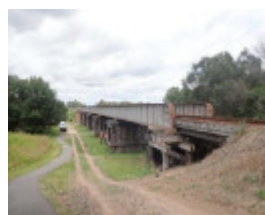
2017, northern approach 1888 section.jpg
