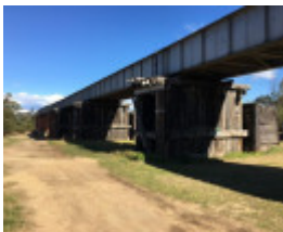
2018 timber piers 1888 section.jpg
