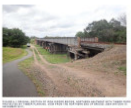
2017, Northern approach, 1888 section .jpg
