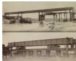
1896 Girders being moved into place with trolleys.jpg
