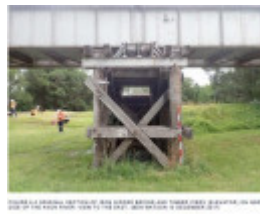
2017, 1888 section, timber piers and iron girders above.jpg
