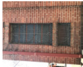
Tapestry brick and window grill
