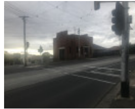
Brunswick West Tramway Substation
