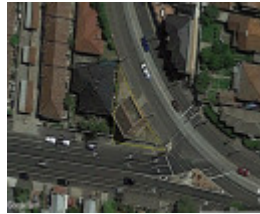
Brunswick West Tramway Substation from above
