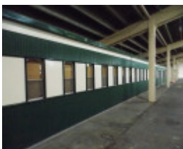
Original tote building in undercroft area north end showing hatch-like windows.jpg
