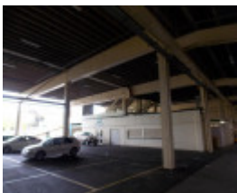
General view of undercroft area showing exposed structure and low-rise infill.jpg
