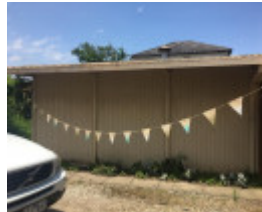
Grant House 2018, West facing elevation (rear module).jpg
