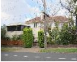
486 Burke Road, seen from Pine Avenue.
