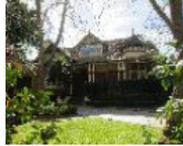
View Street 15 (2).jpg
