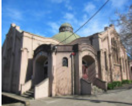
Canterbury Road, 146 CANTERBURY PRESBYTERIAN CHURCH
