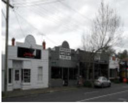
Canterbury Road, 351-359 VICTORIAN SHOPS
