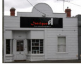
Canterbury Road, 351-359 VICTORIAN SHOPS
