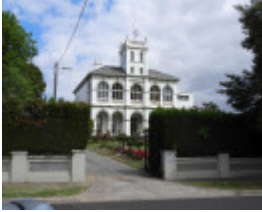
Aberfeldie Street and Waverley Street Precinct
