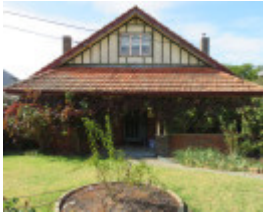
16 Ballater Street Essendon
