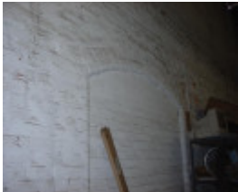
Segmental arched opening in south wall
