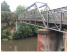
Walmer Street Bridge - view from south bank - 2019
