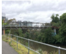
Walmer Street Bridge - 2019
